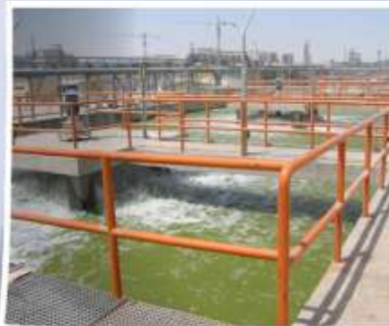
Industrial wastewater treatment
