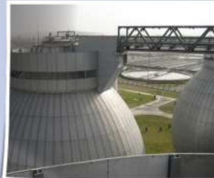
Sewage sludge treatment
